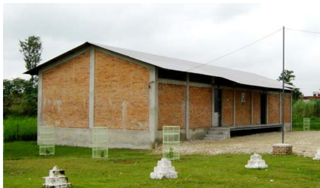
Newly constructed district store in Parsa district.
